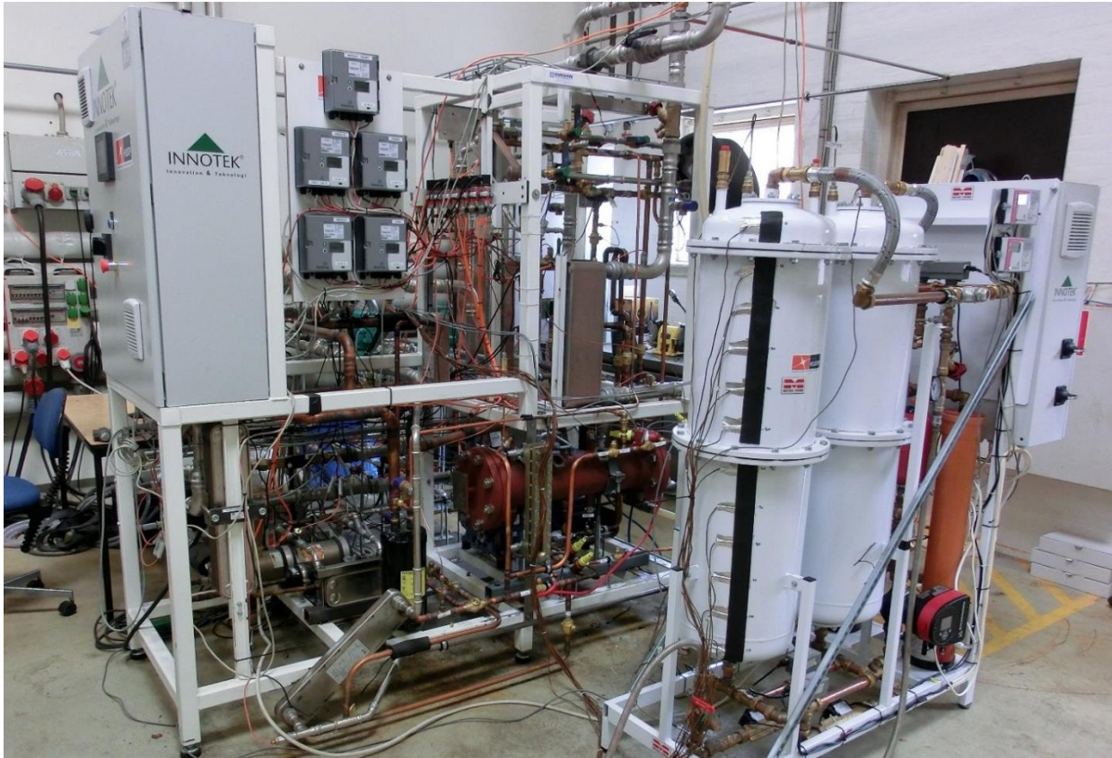
Figure 27 - Storage tank test setup with two storage tanks, a heat pump and a control system.
