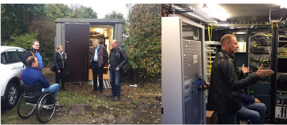
Figure 33 Billund system site with 5kW system in parallel with 3,2kW system and Master controller installed in a old shelter with integrated H2 bottle rack mounted outside..
