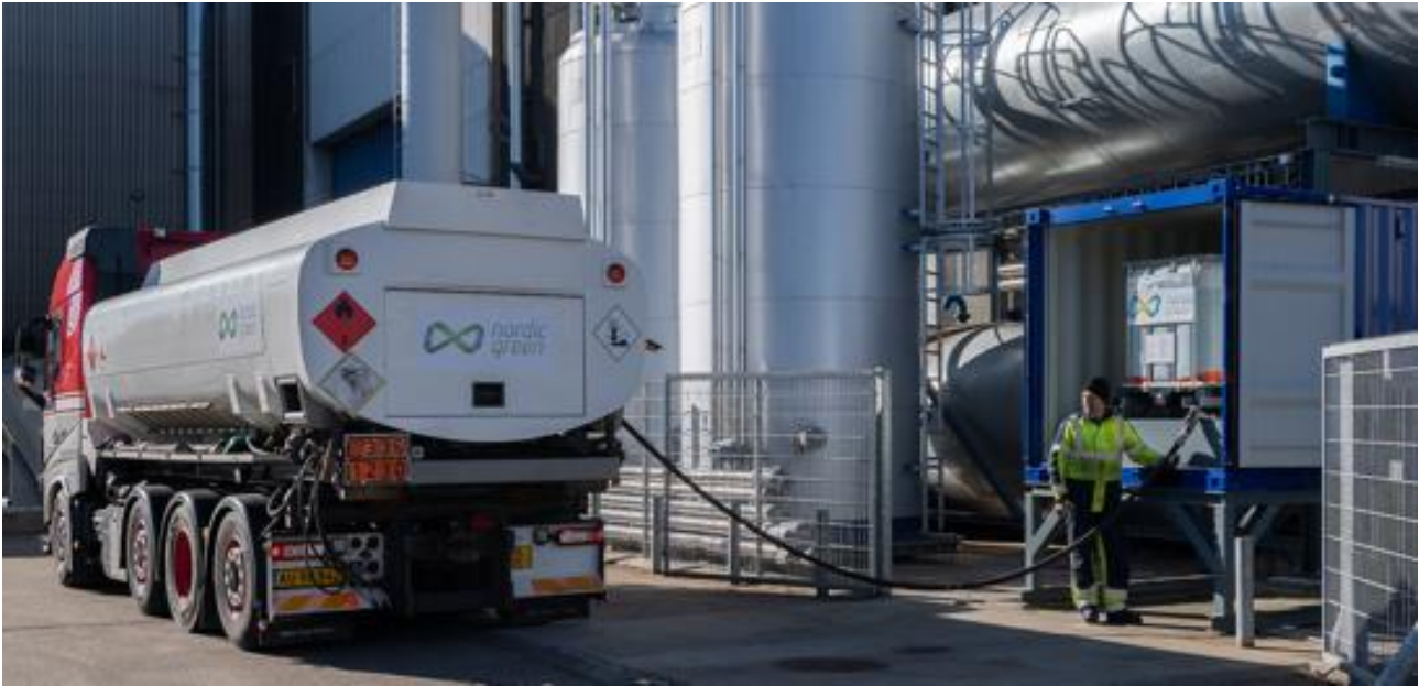
Figure 4 Filling the methanol tank at Alfa Laval Aalborg
