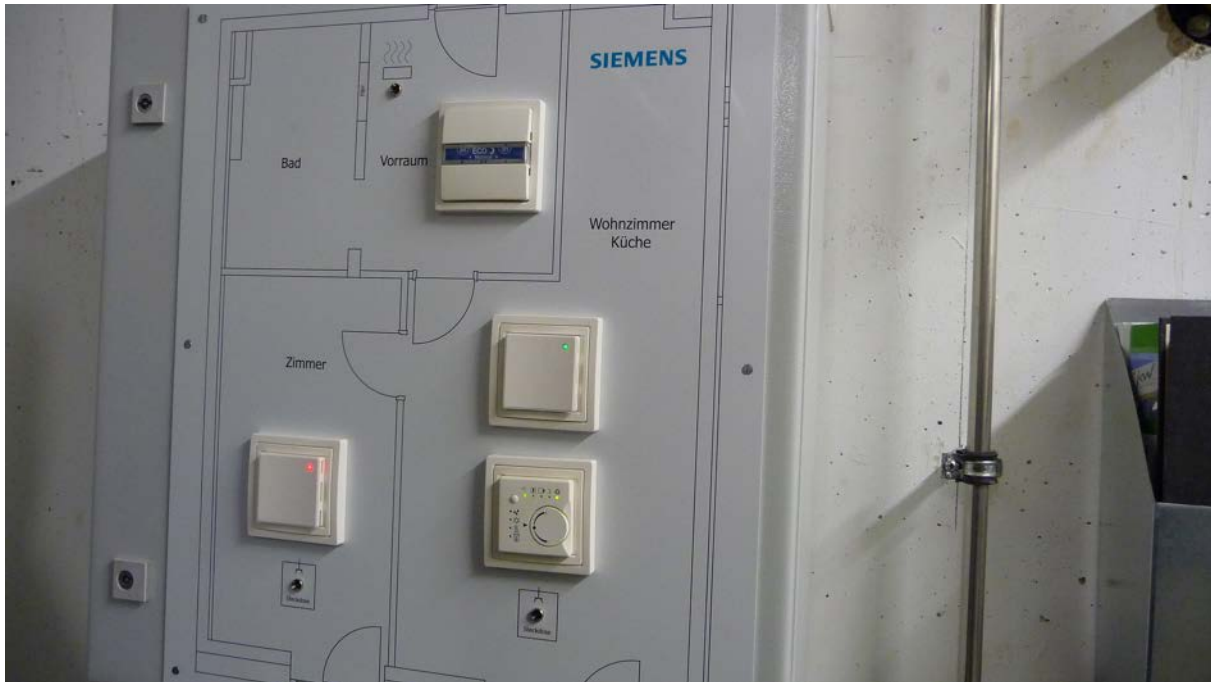
Figure 18: Model of the monitoring equipment switches installed in the monitoring apartments during the field-test
