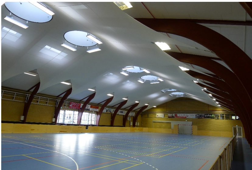
The main hall (this is the old, now refurbished, hall). Notice the natural lighting from above.
