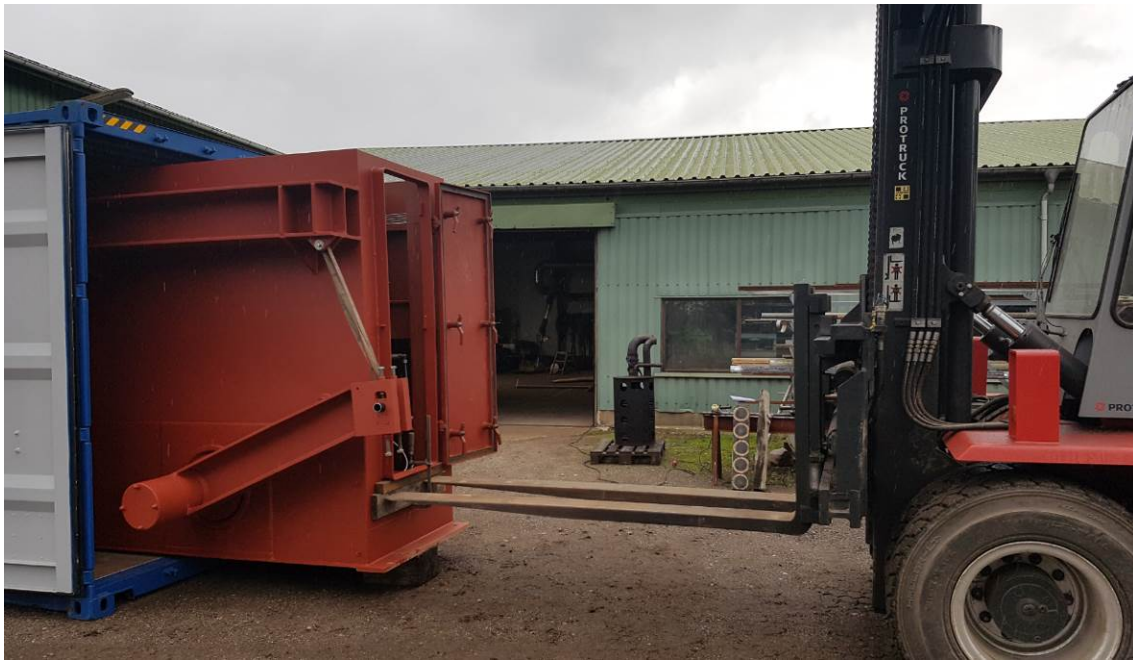
Figure 4. The modified and repainted PTO house are being pushed into the container.
